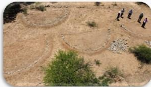
The SLM activities include the construction of half-moons
